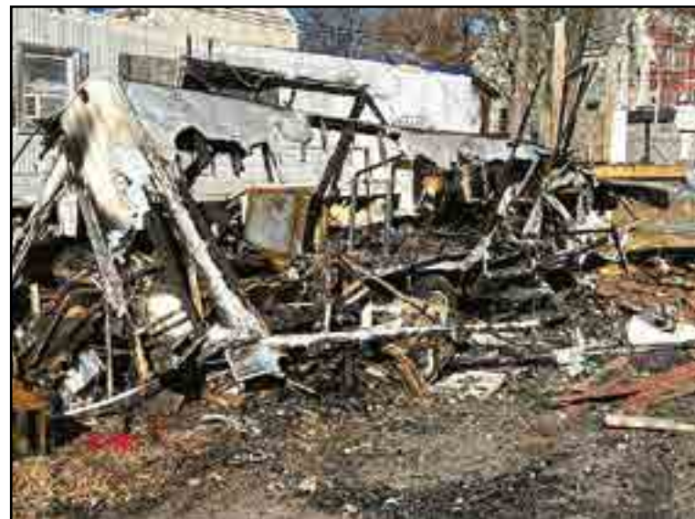
This is the aftermath of a fire that destroyed this mobile home at the former Lee's Trailer Park.
